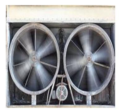
"Mechanical" or "forced" ventilation is provided by an <u>air handler</u> and used to control <u>indoor air quality</u>. Excess <u>humidity</u>, odors, and contaminants can often be controlled via dilution or replacement with outside air. However, in humid climates much energy is required to remove excess moisture from ventilation air.
